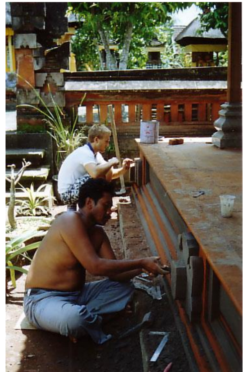
Second year architecture student David Mitchell (background) learning to carve local siltstone on the face of a Bale Gede in the studio compound.
